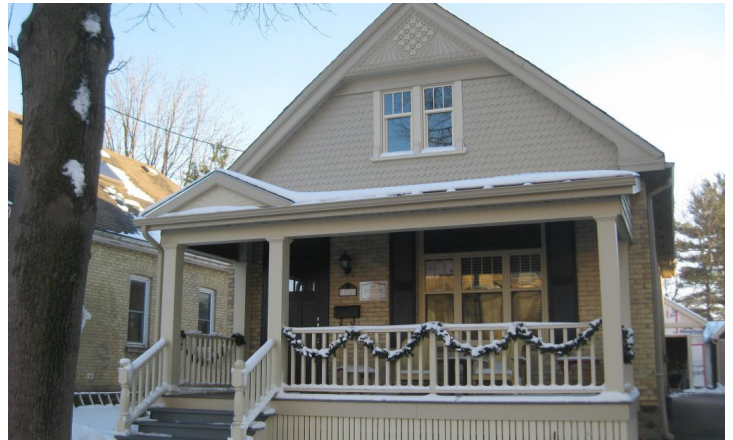
135 Duchess Avenue - completed
